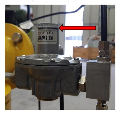
• Check the perfect condition of the internal seal and replace it if necessary
